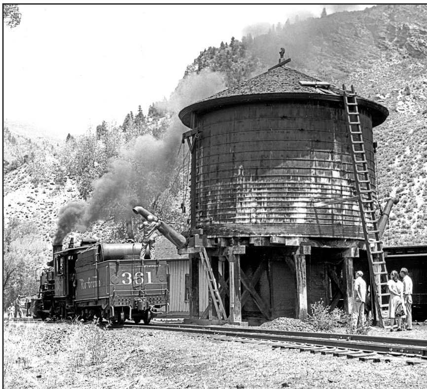
D&RGW engine 361, a 2-8-0, originally Crystal River RR No. 102, Baldwin 1900, acquired by the D&RG in 1916. These locomotives sometimes were referred to as "Little Mudhens." This engine was dismantled at Pueblo on November 15, 1951. This scene is at Cimarron taking water prior to train returning to Gunnison. – Jack Pfeifer photo from the James L. Ehernberger collection.
